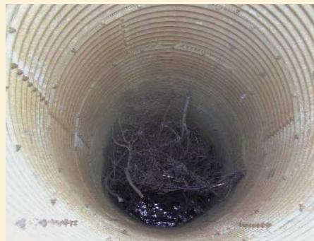
Abandoned well contaminated with UXO
